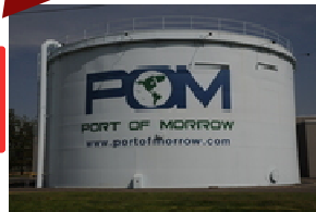
Not far from this water tower in Boardman, Ore., construction has begun on a data center for Amazon.
